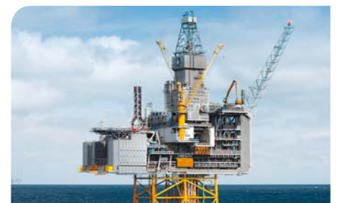
LM gas turbines offer high reliability, which makes them the ideal choice of power plant for use on oil rigs.
